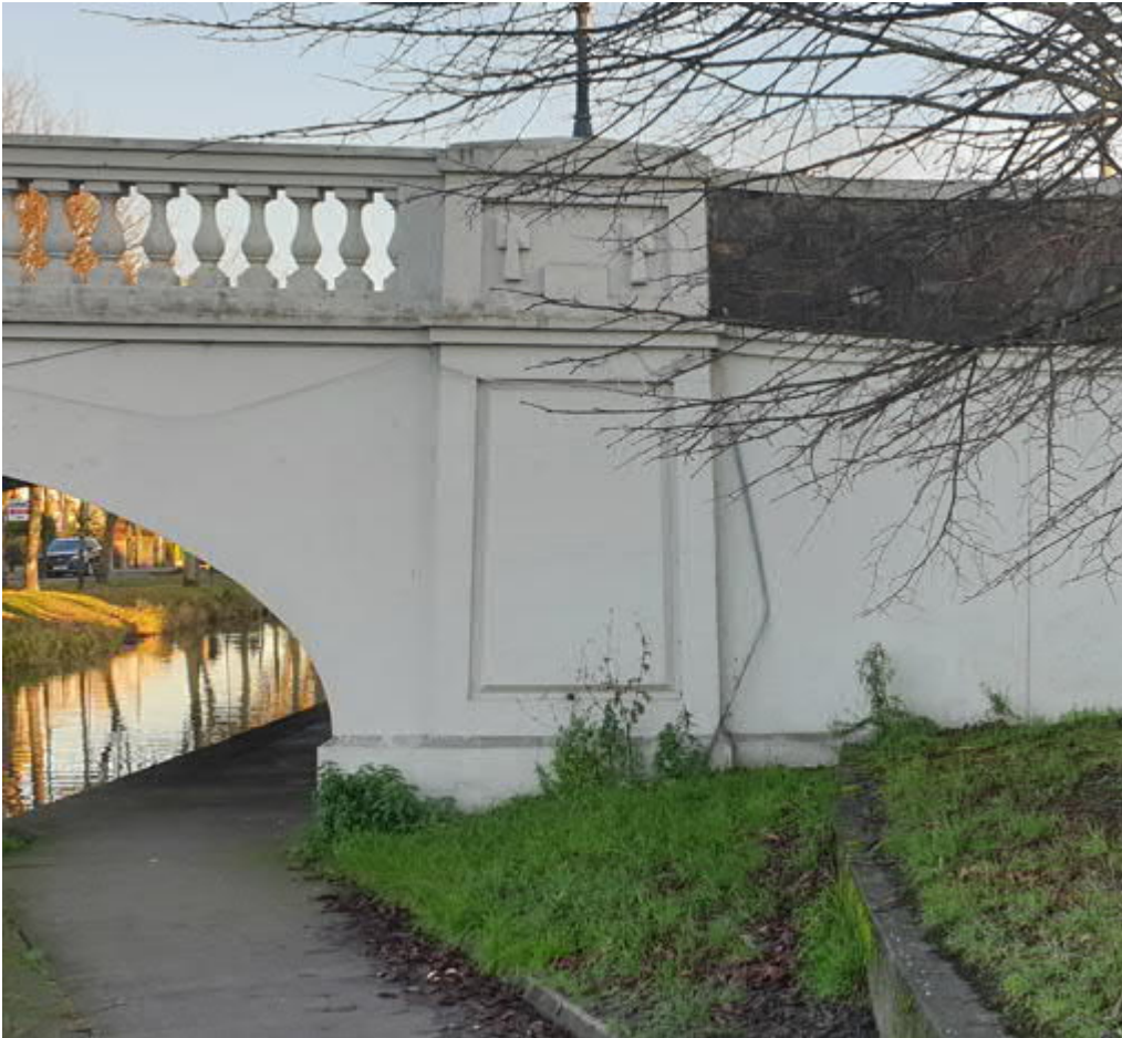
Figure 7: Bridge foundation and clearances
