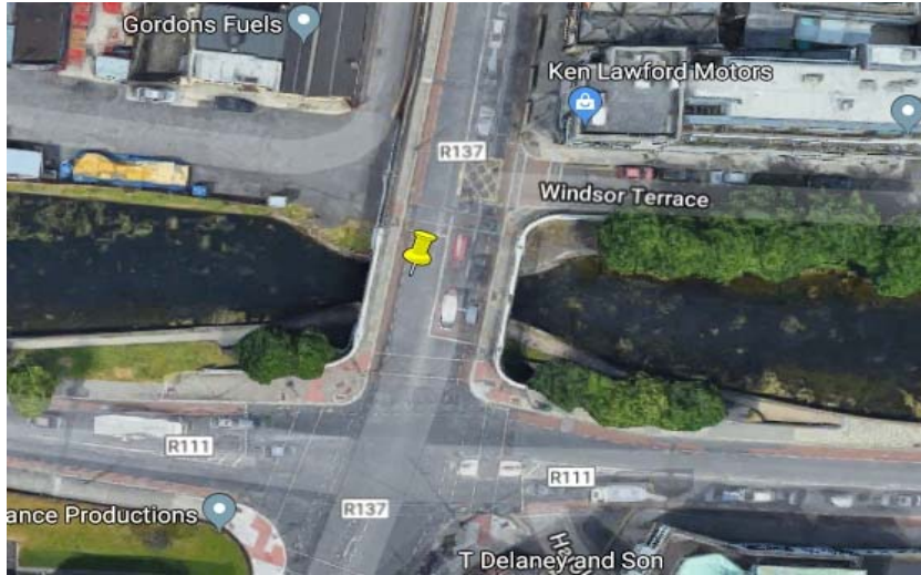
View from south abutment
