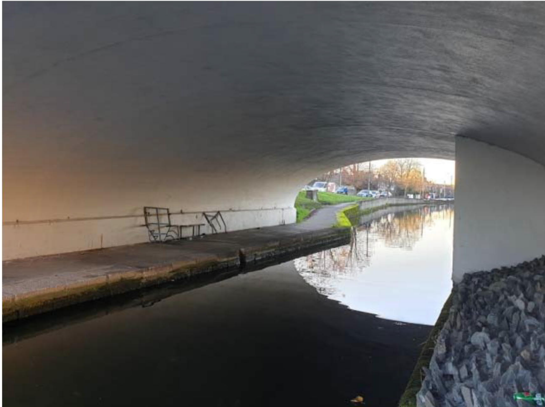
Figure 5: Soffit of Harold Cross Bridge / Robert Emmet Bridge
